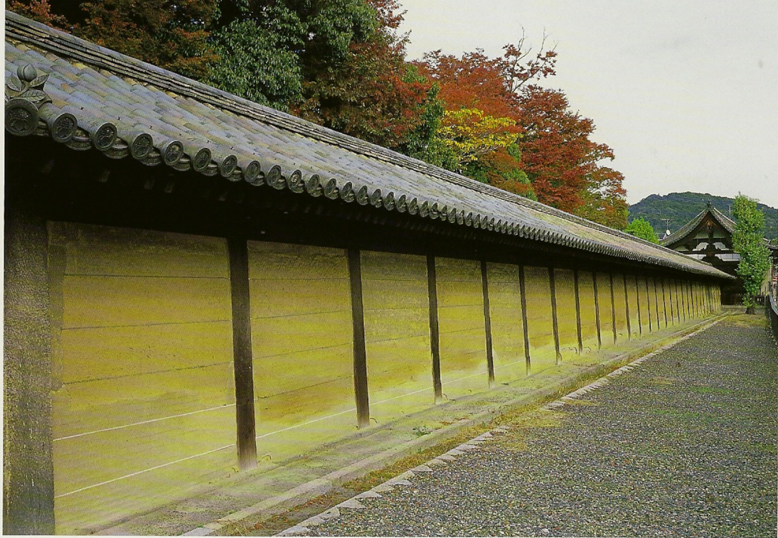
Taikou-bei : Earthen wall (Important cultural property : Momoyama period)
